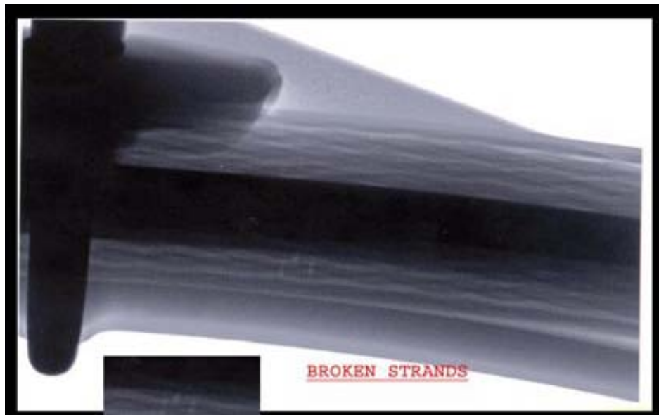
Broken Strands inside standard suspension clamp. X-Ray Photo Courtesy USAirmobile
