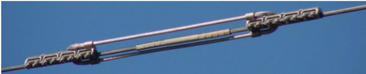
Photos of the splice below have the characteristics typical of “single die” connectors, being the “short” un-crimped section in the center and crimped with a type CD “round die” as opposed to hex dies.
