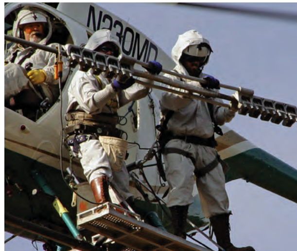
Linemen position the ClampStar mid-span shunt around the 1590 kcmil 54/19 ACSR single-die compression splice.
