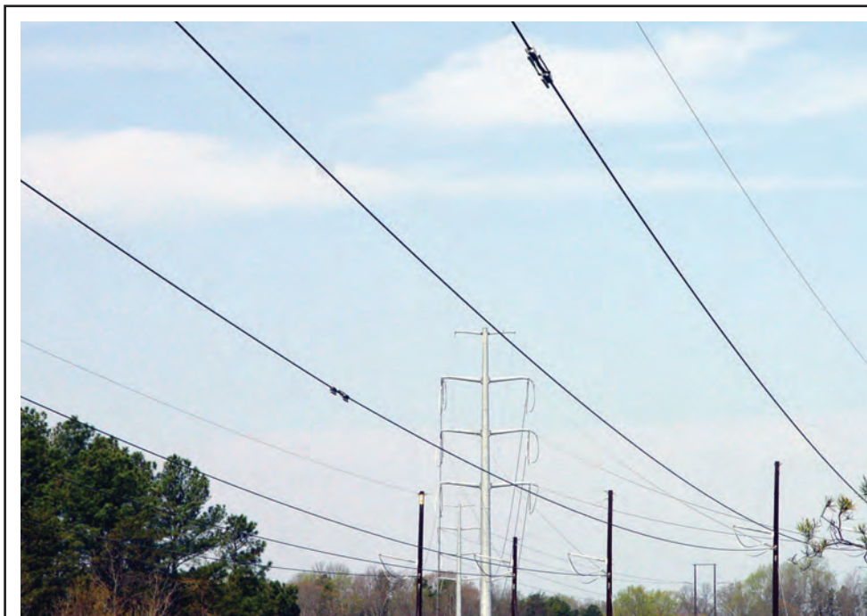
The transmission lines run horizontal out of switchyard for several spans then roll to the self-supporting, single-pole structures shown in the background. The installed ClampStar mid-span shunts are shown on the conductor.
