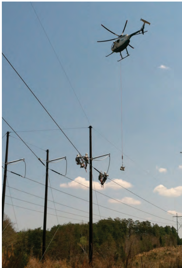
AIR2 helicopter crew performs work on dead-ends.
