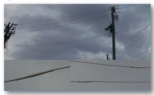
These are definitely "installation errors" or more appropriately "application errors" where the wrong device, in these examples an automatic splice, should never have been installed.
