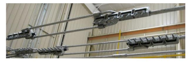
The intended application of ClampStar® is a "Connector Corrector" to be installed over a connector, or a damaged section of a conductor in normal tension. Thus, initially installed, there is no tension on the ClampStar, just as there is no tension imparted to trousers on a clothesline.
